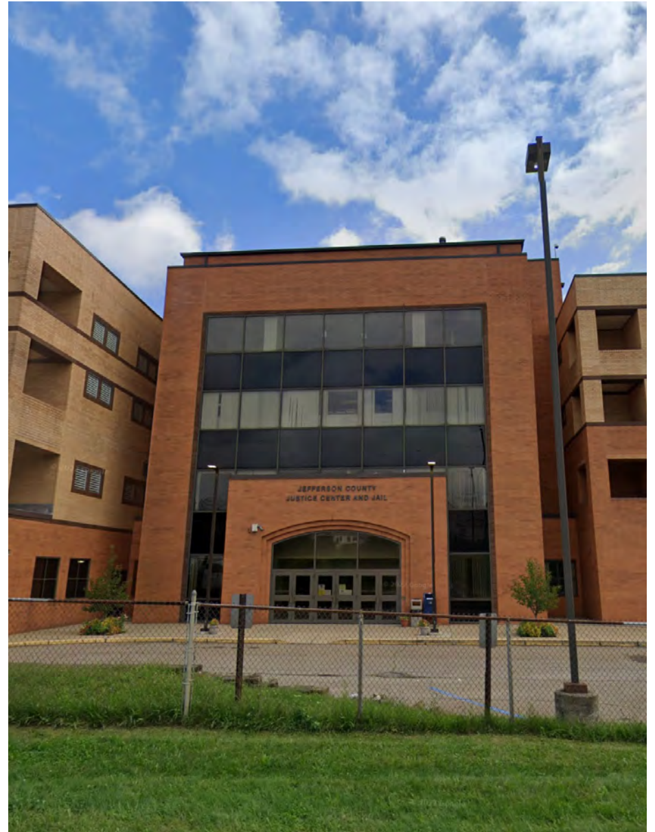
Jefferson County Justice Center and Jail
